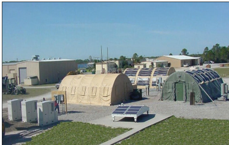
Figure 4: Renewable Energy Tent City at Tyndall Air Force Base, Florida
