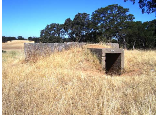
Existing bunker used as vertical control structure
