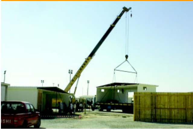
Civil engineers at Al Dhafra found that the most efficient way to erect buildings in that area of the world was to purchase modular ones and have them delivered to the site.
