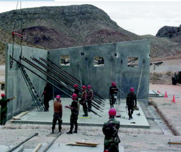
820th RHS members used the tilt-up method to construct a quarry maintenance facility on Nellis AFB. (Photos courtesy 820th RHS)
