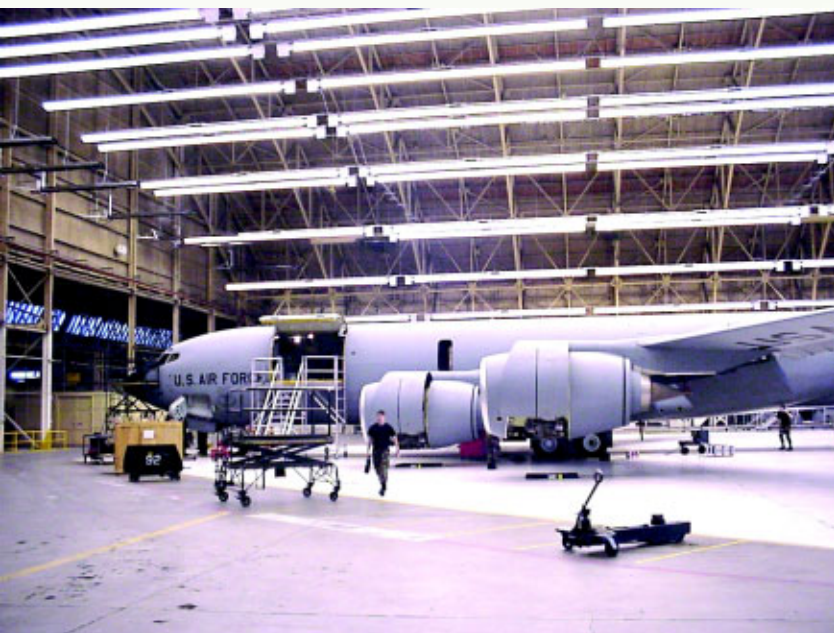
There is literally a “day and night” difference in the new and old lighting systems in the hangars. Photos show Hangar 1 (above) with light pipes installed and Hangar 4 (left) with the old pendant light fixtures. (Photos courtesy 92nd CES)
