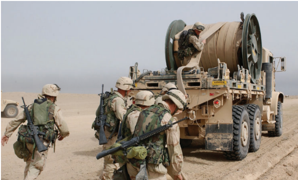
Figure 3.1 U.S. Marine Corps Hose Reel Conduit Being Emplaced in Iraq
