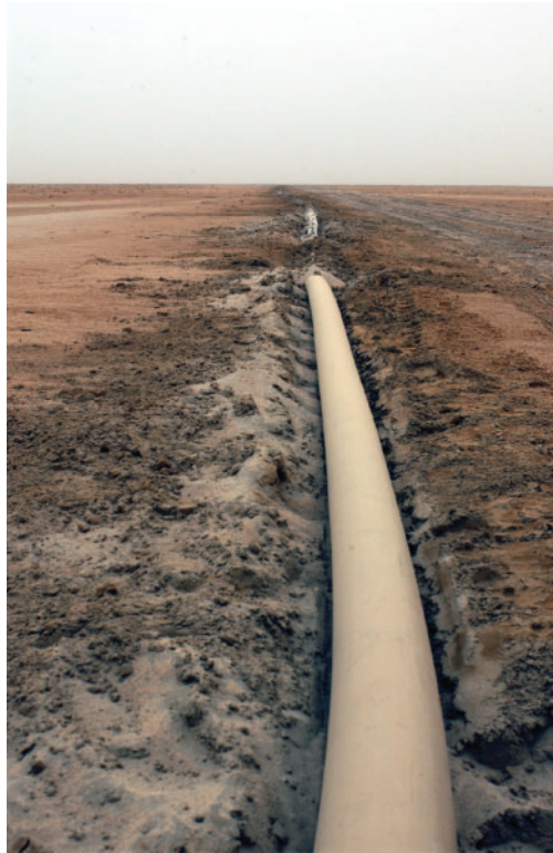
Figure 2.2 HRS Laid in V-Shaped Ditch in Southern Iraq
