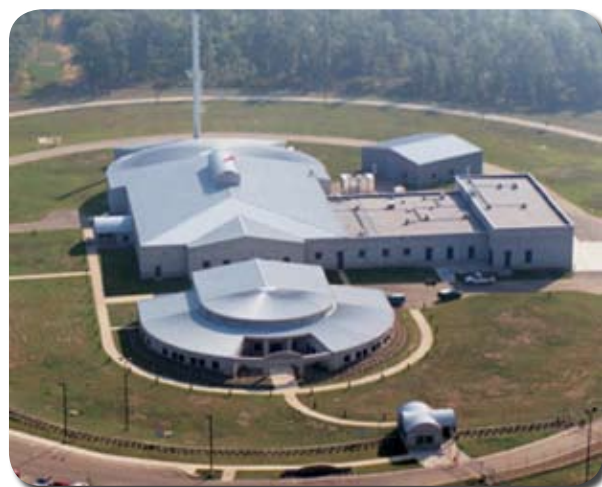
Figure 4-1. Chemical Defense Training Facility (CDTF)
