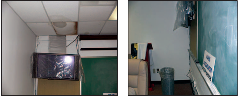
Figure 5: Damage from a Leaking Roof at the Public Works Building at Naval Air Engineering Station Lakehurst
