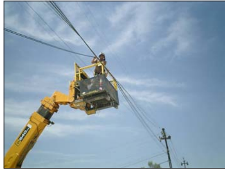
(Above) SGT Steve Achten Delta Company, 29th Signal Battalion installs aerial fiber at FOB Marez.
