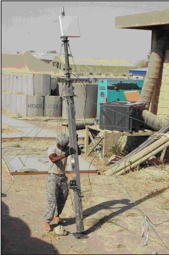
(Left) SGT Karl Vinson, C BSTB/3IBCT/25ID, hoist an antenna mast with an OS Spectra: ODU mounted on it. SGT Daniel Thompson
