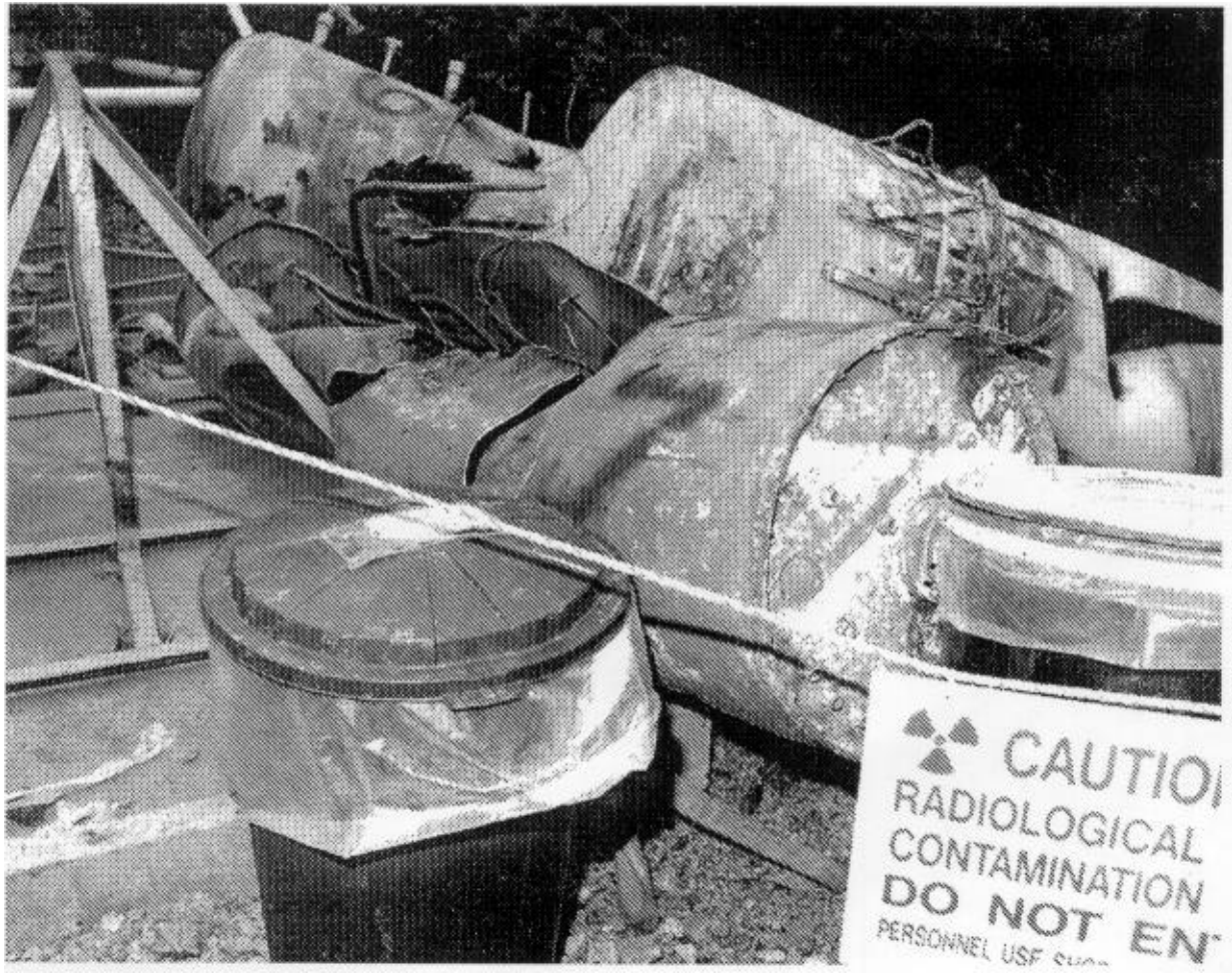
VIEW OF VESSELS EXPLOSIVELY BREACHED (Fig. 6)
