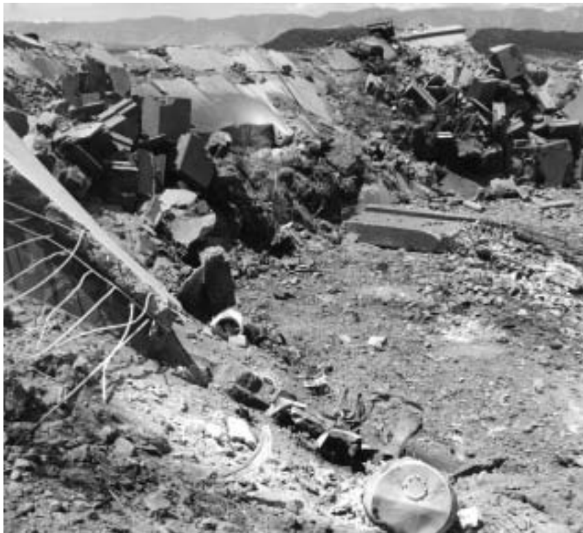
Figure 22. View of CT1 structure taken from 90° azimuth.
