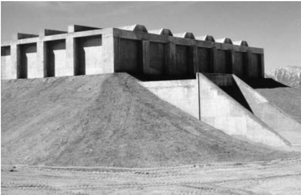
Figure 10. Exterior view of CT1 structure.
