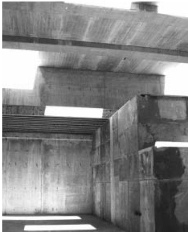
Figure 12. Portion of aisle wall.
