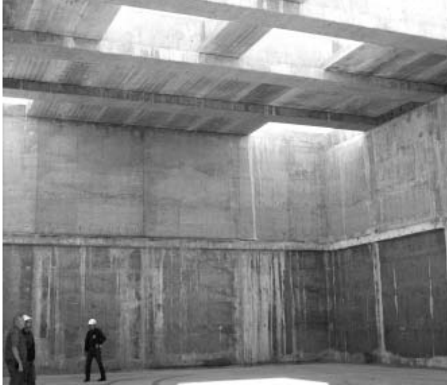
Figure 11. Interior view of CT1 structure.
