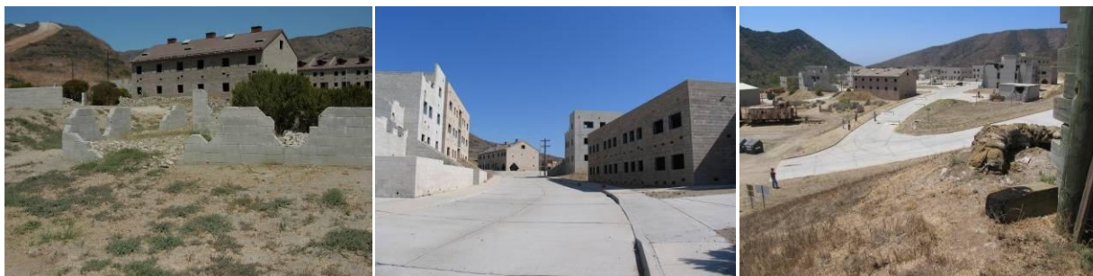
Figure 1. MOUT test site at Camp Pendleton consists of multiple buildings and varying terrain.
