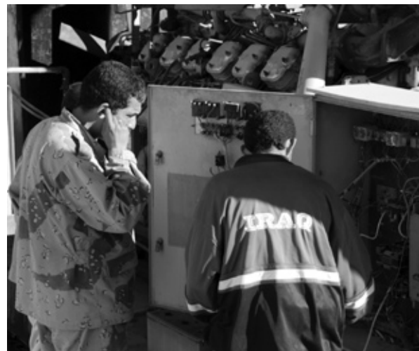
Iraqi municipal workers work on a generator in a sewer water lift station during Operation Al Fajr, November 2004.
