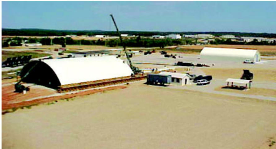
The new 366th TRS, Det. 7 training complex is the handiwork of several different civil engineer units. Shown here is the pre-engineered classroom building (left, rear), the 45' by 110' Ultimate Building (right, rear), and the 80' by 200' Super K-Span building at the halfway mark in construction (left, front). (Photo courtesy 366th TRS, Det. 7)
