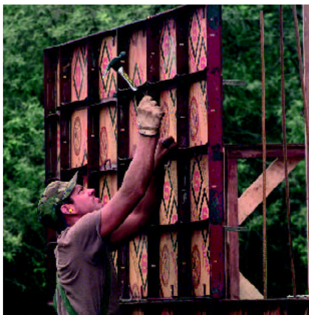
(Right) SSgt John Carter, 819th RHS, hammers a nail into the forms for the wall structure of a two-room school in Camatindi, Bolivia. (Photo by TSgt Katherin D. Bryson)
