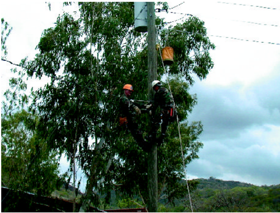
SMSgt Tommy Guerra, 144th CES, and SSgt Rex Rekow, 142nd CES, install a secondary feeder to the billeting area as part of the complete rewiring of the secondary distribution system for the base camp.
