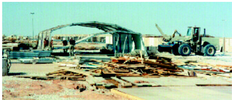
Structures specialists from the 49th Materiel Maintenance Group disassemble a General Purpose Shelter for relocation to the new Friendly Forces Housing Complex at Prince Sultan AB.
