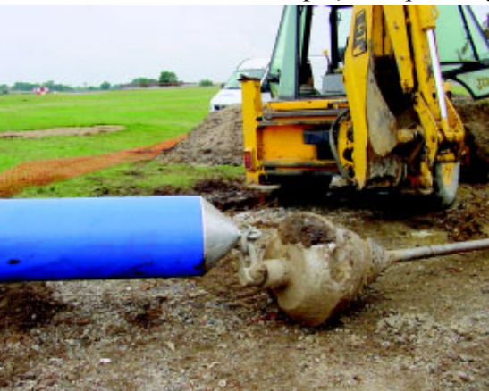
Directional drilling uses a system of augers, pipes and Bentonite clay material to install pipe with little outward disturbance.
