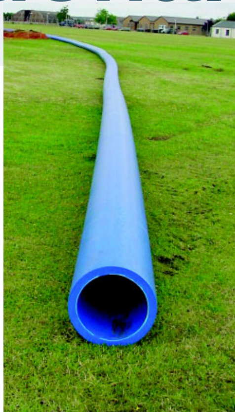
The Lakenheath project required installation of over 13 miles of 16-inch internal diameter high-density polyethylene pipe around the bases runways and high-traffic areas. (Photos courtesy 48th CES)
