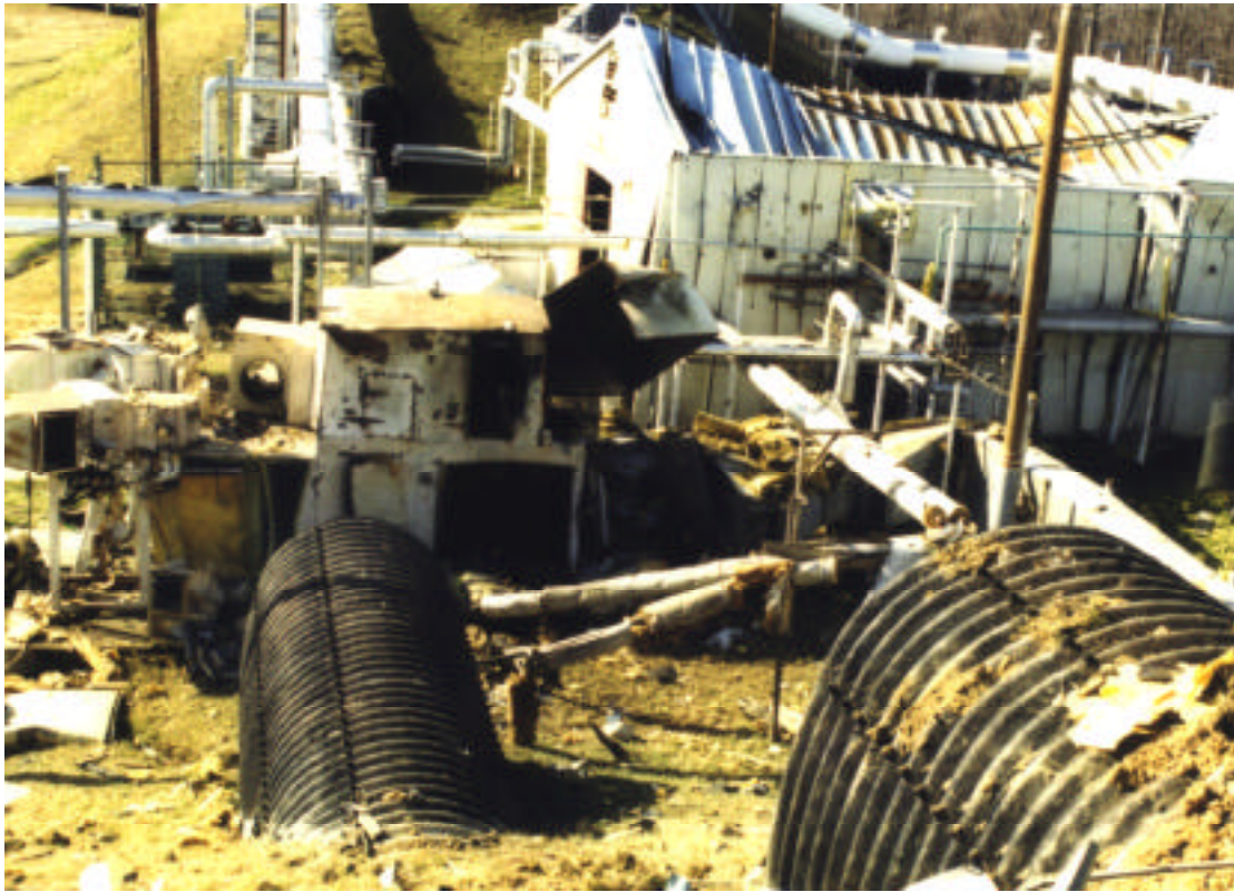
FIGURE 6. VIEW FROM TUNNEL ENTRANCE
