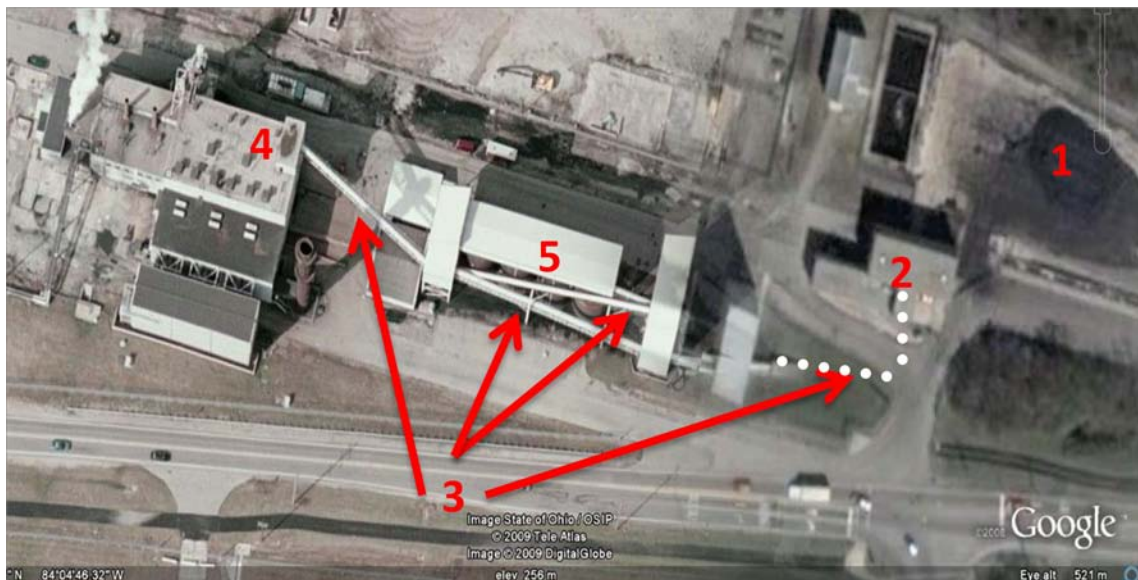
Figure 2: Building 770 Heat Plant Area B (Google, 2009)
