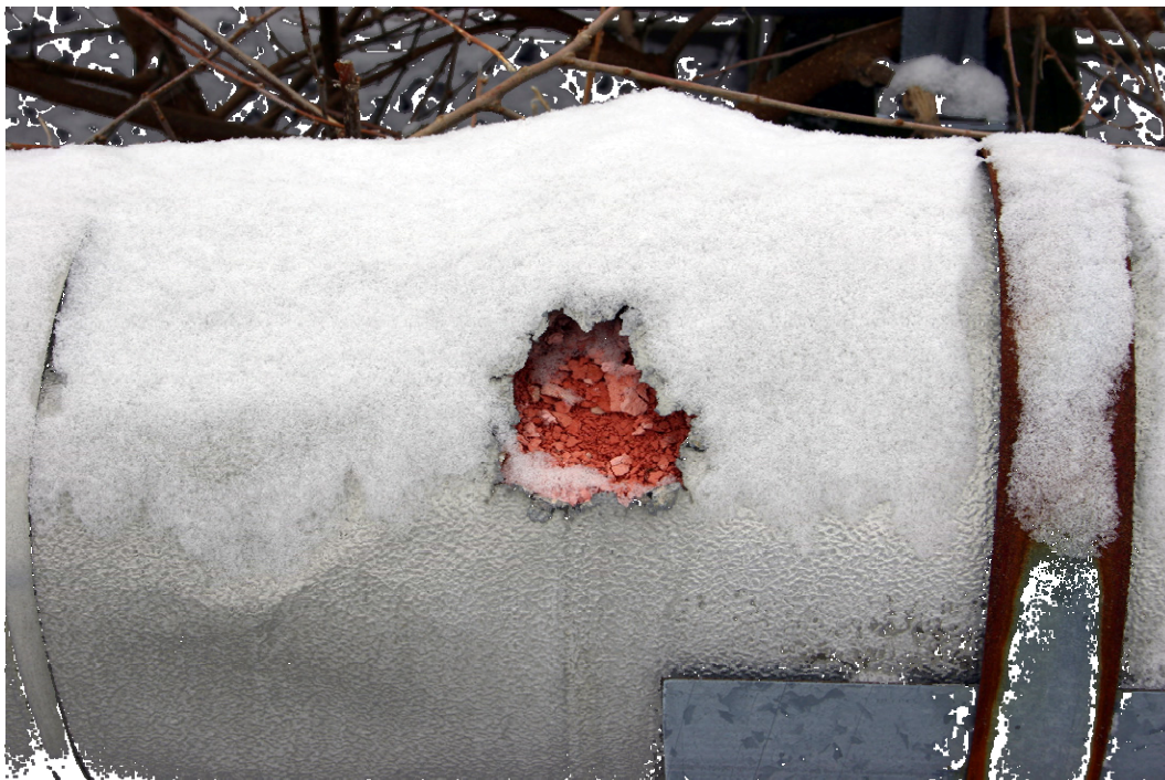
Figure C6. Photograph of another hole in aluminum weather cover on the header.
