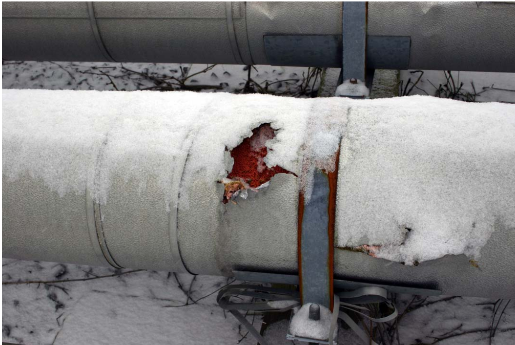
Figure C5. Photograph of another hole in aluminum weather cover.
