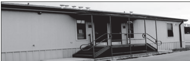
Source: GAO. Barracks at Fort Hood, Texas.
