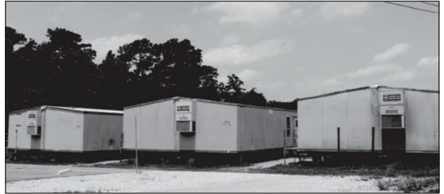
Source: GAO. Administrative space at Camp Lejeune, North Carolina.
