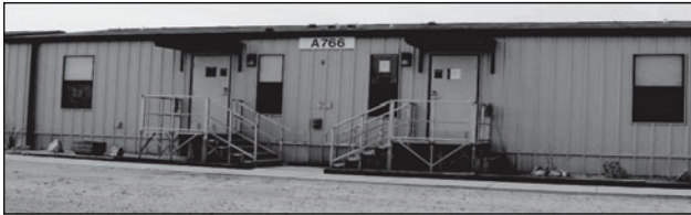
Source: DOD. Barracks at Fort Bliss, Texas.
