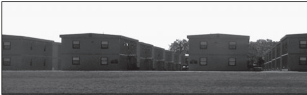
Source: GAO. Barracks for about 600 soldiers at Fort Drum, New York.
