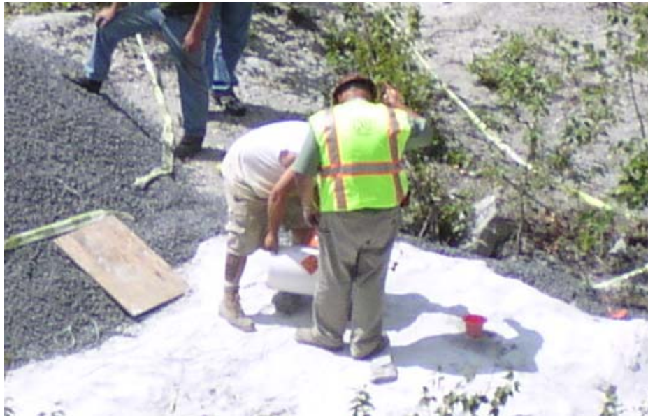
Figure 63. Loading of ANFO/Emulsion explosive.
