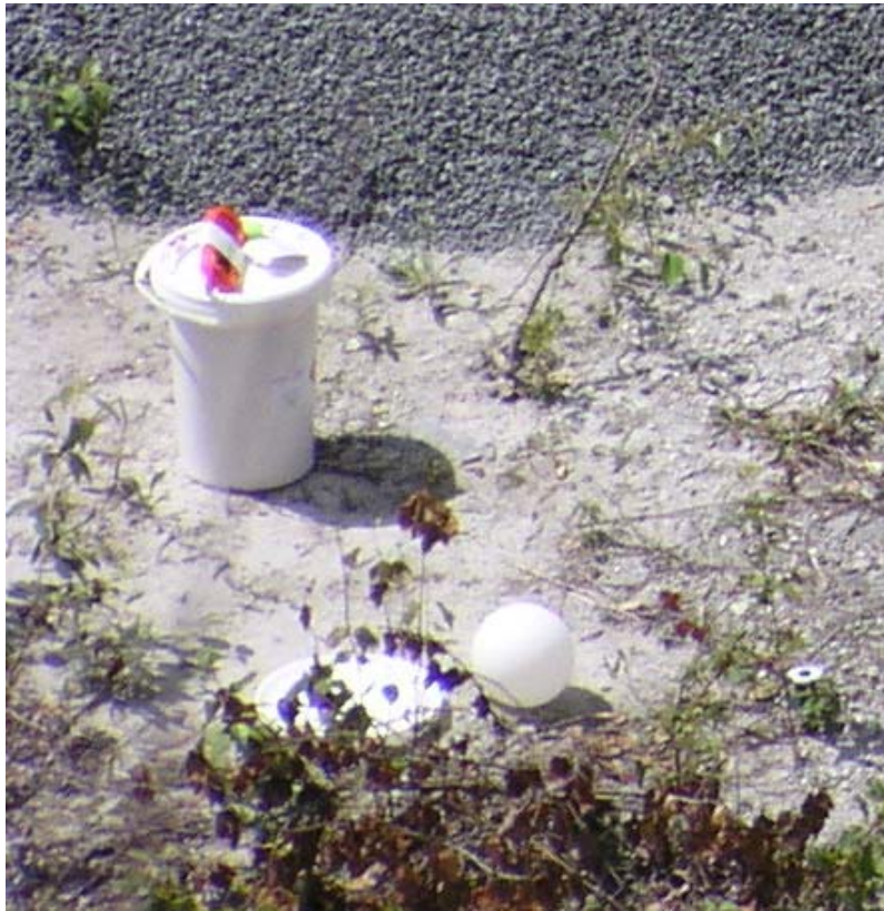
Figure 66. Blast plug (white ball) used to help stem the holes.
