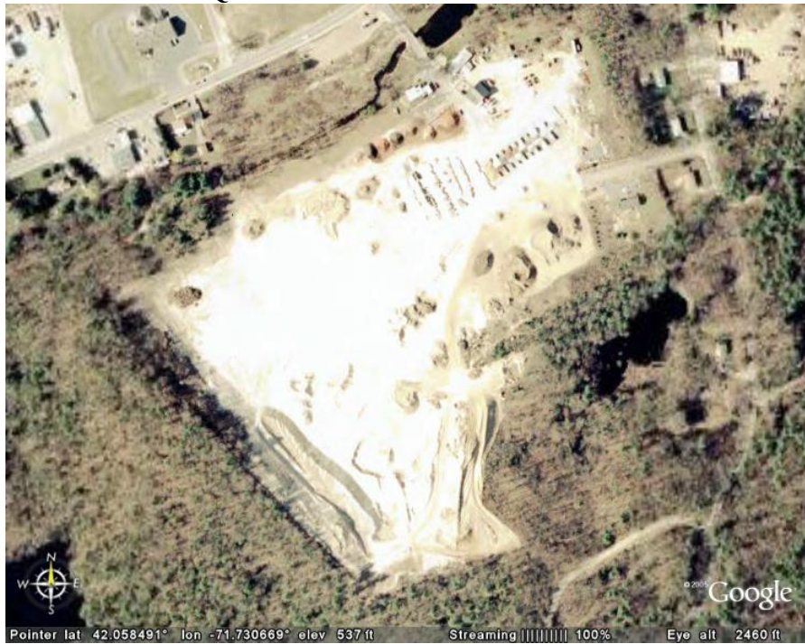
Figure 13. Percy Guiou Excavating, Douglas, MA – Photo from Google Earth
