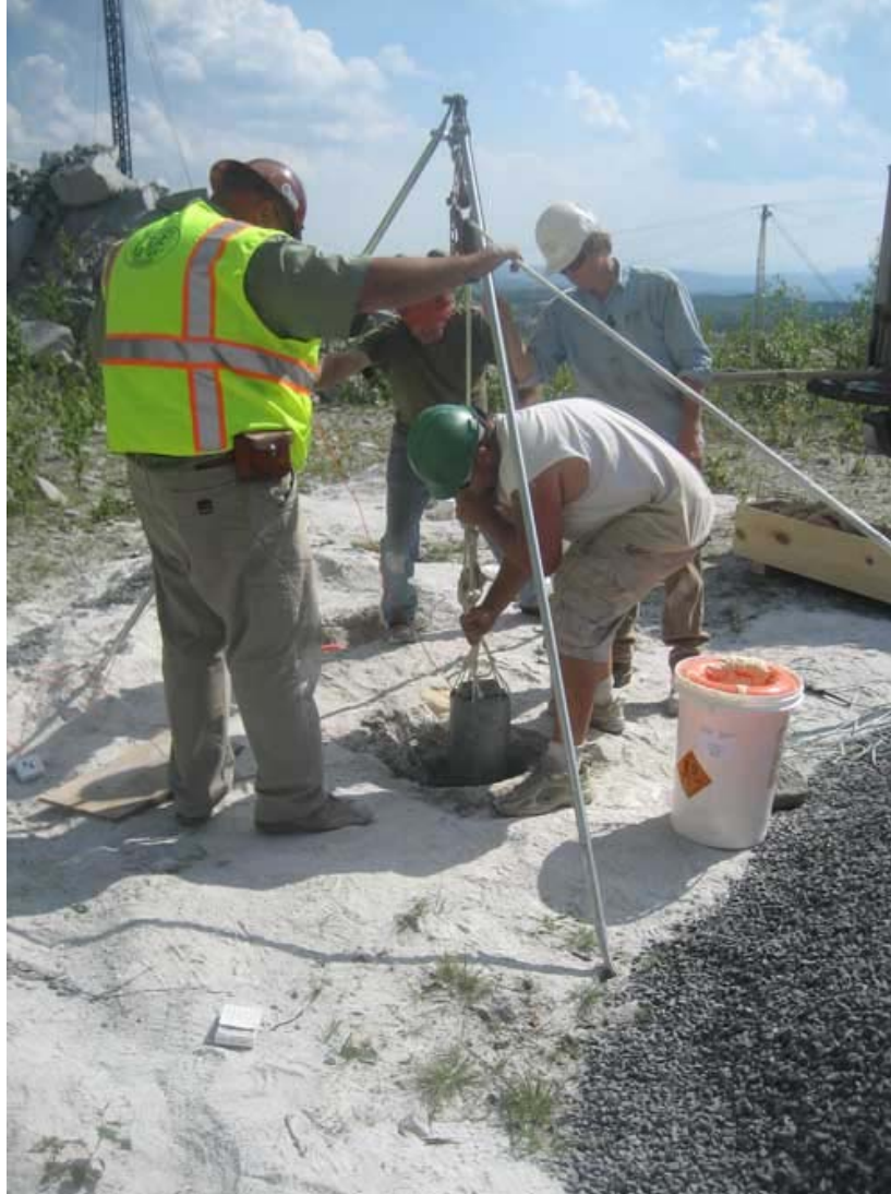
Figure 65. Lowering the COMP B charge into the hole.
