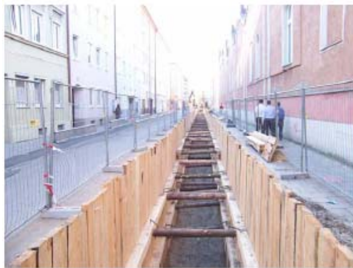
Figure 7.3. Trench/canal for a buried pre-insulated pipe.
