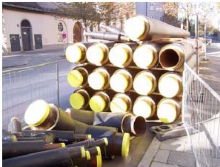
Figure 7.4. Pre-cast fittings and elbows of pre-insulated bounded pipes.
