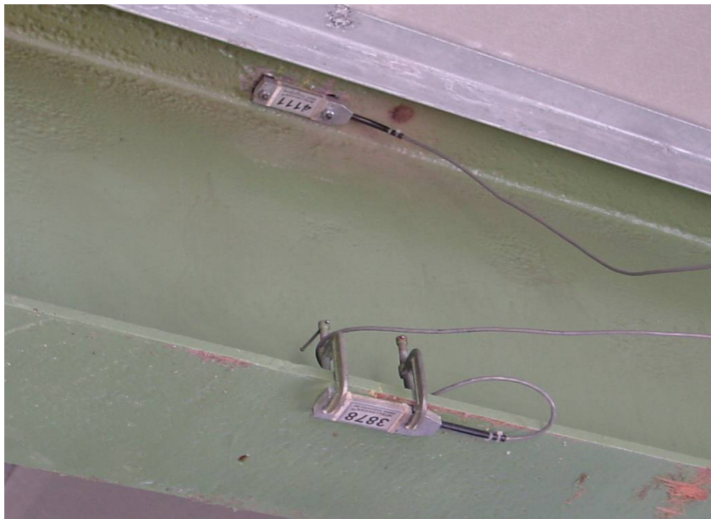
Figure C1. Strain transducers mounted on a steel girder.
