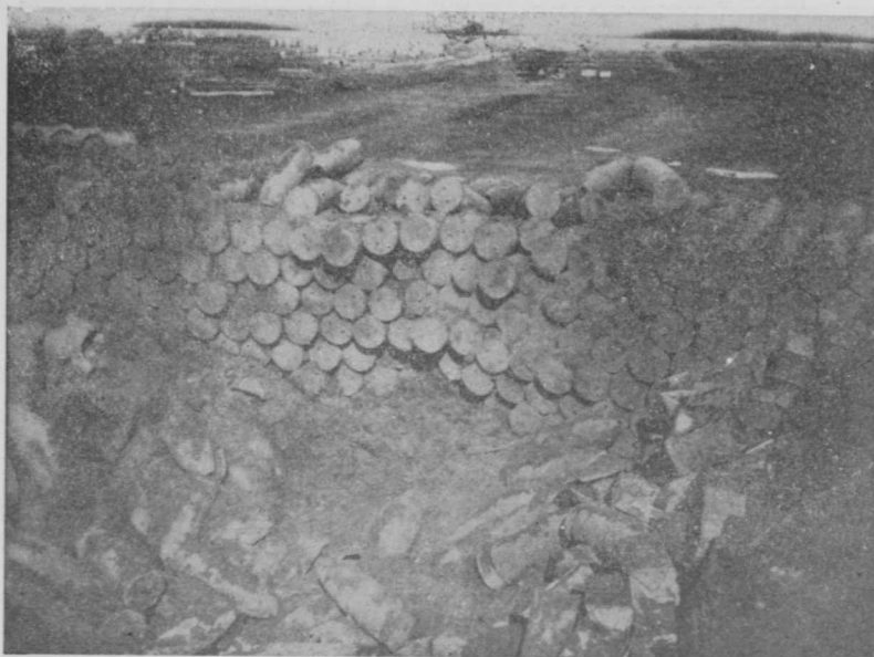
FIG. 7. 9.2-INCH LYDDITE-FILLED SHELLS IN CUBICLE Explosion caused by absence of tanks filled with water
