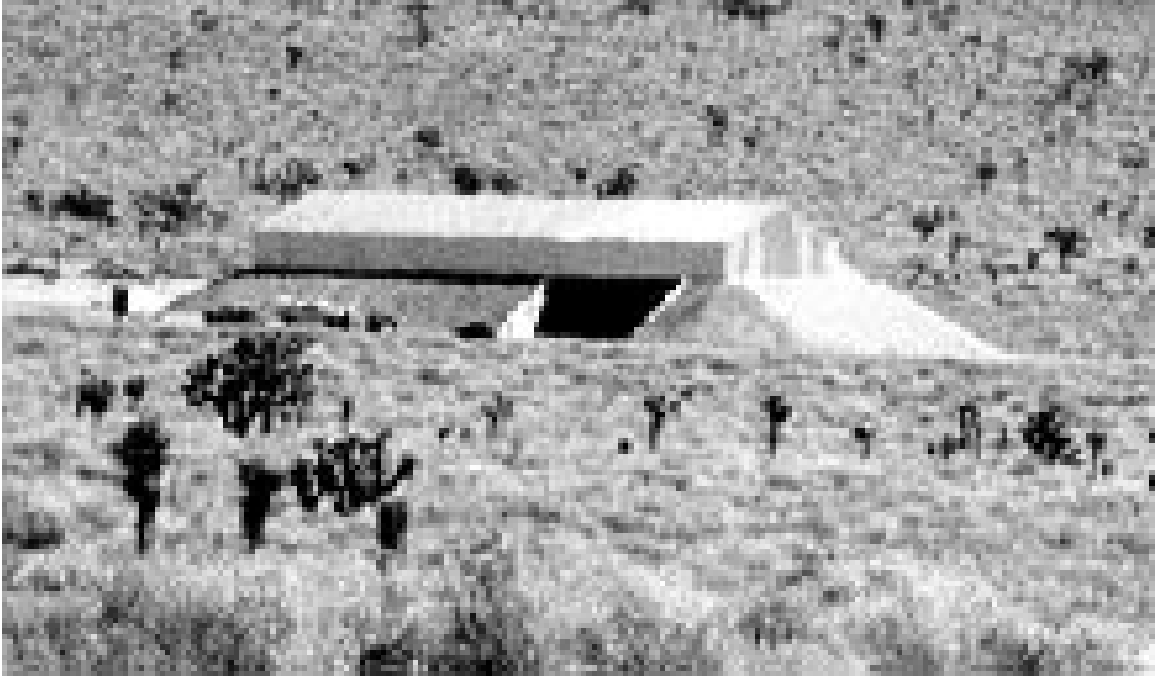
Figure 9. Exterior view of CT3 structure.
