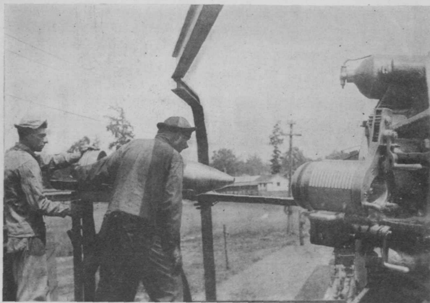
CUT DOWN TILTED TRAY AND GRAVITY LOADING FOR 12-IN. RAILWAY MORTARS
