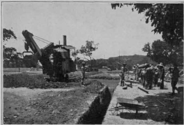
Excavating for the Corregidor Club Swimming Pool.
