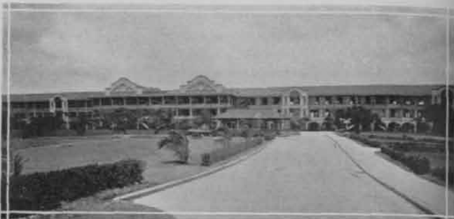
Topside Club, Showing Recently Completed Parking Space.
