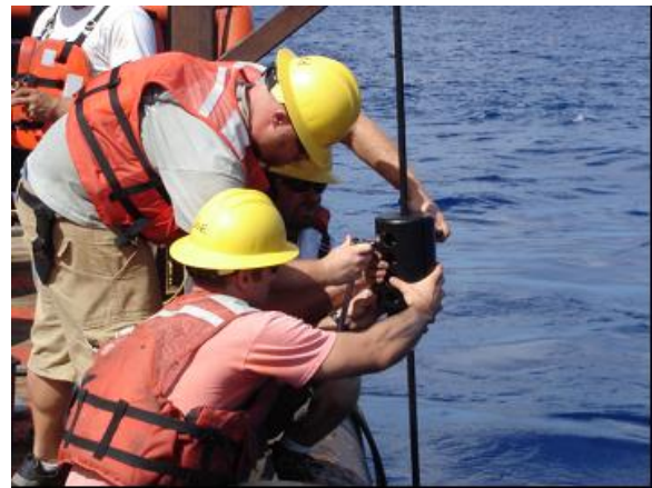
Figure 43 Bolting Cable Stopper to the Counterweight Cable
