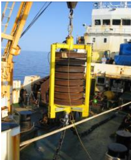
Figure 8 Main Mooring Clump Anchor
