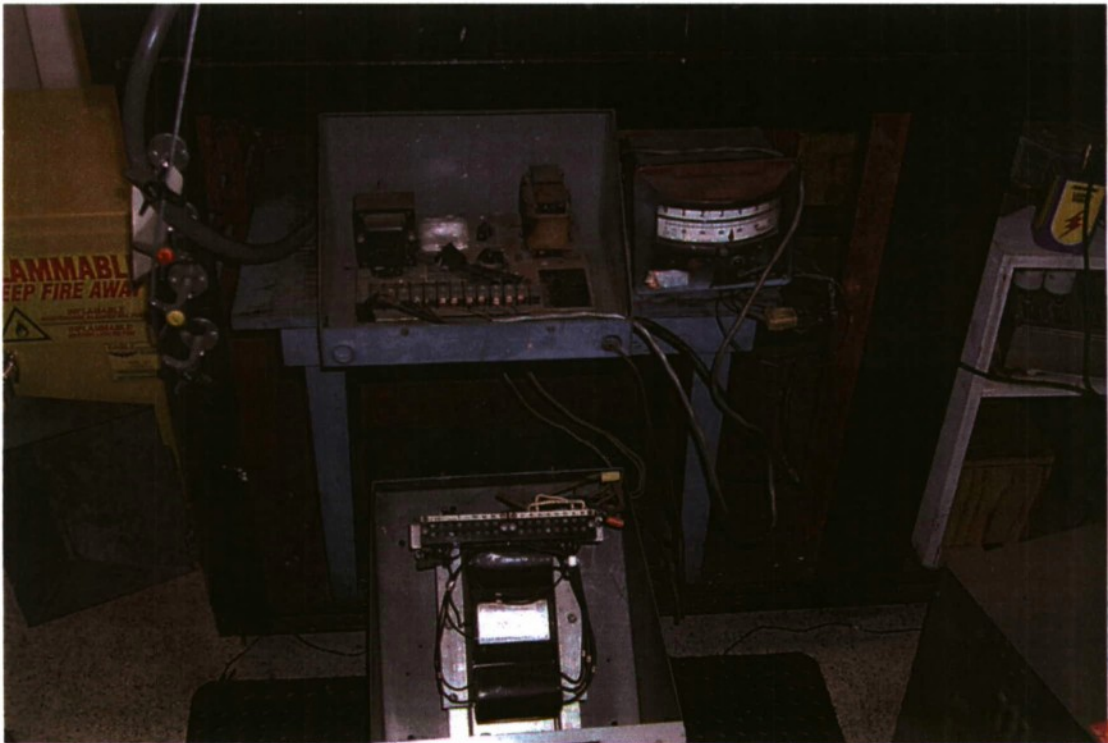
Figure 1 West controller and saturable reactor
