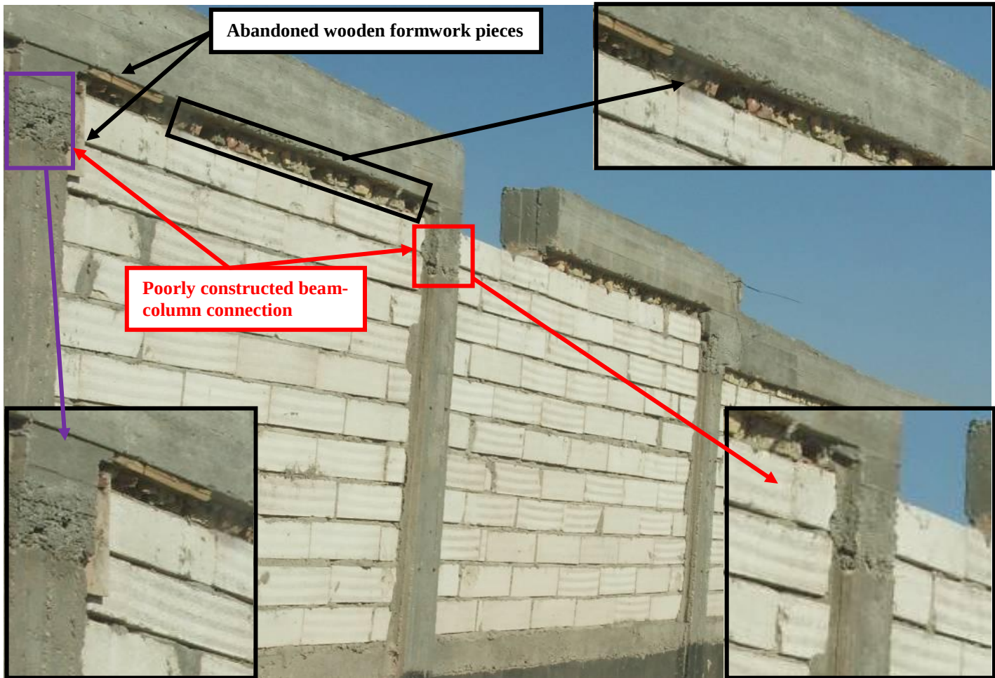
Site Photo 3. Perimeter security wall construction
