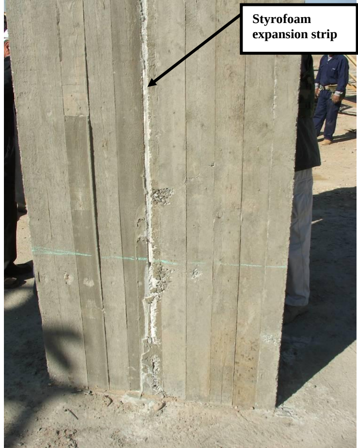
Site Photo 15. Example of Styrofoam expansion strip
