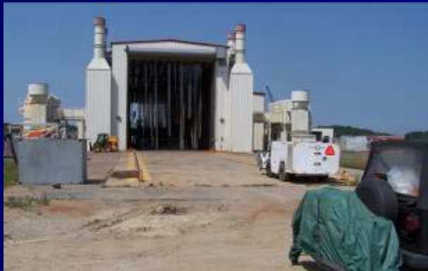
Bridge Caisson Maintenance Area
