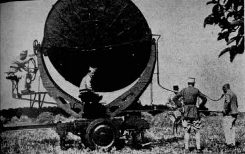
Left: FRANCE—A parabolic sound locator used at the 1936 air maneuvers.
