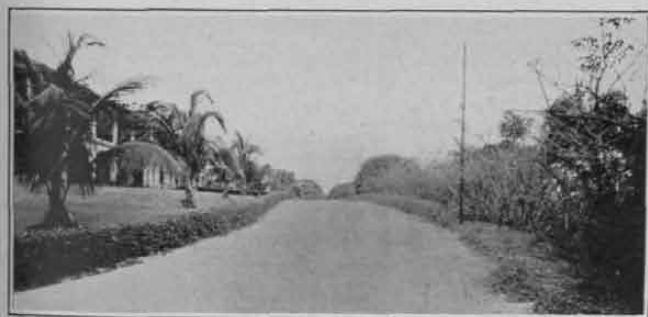
New Asphalt Road Around Hospital.
