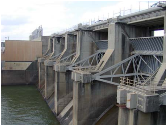
Figure 7. Tainter gates and trunnions.
