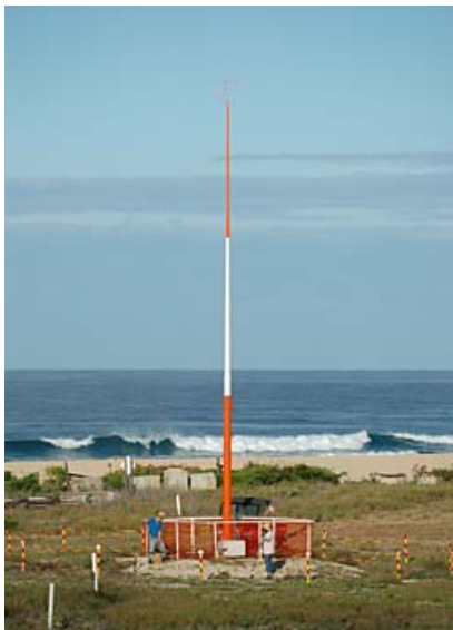
Figure 10. WWVH 10-MHz antenna.
