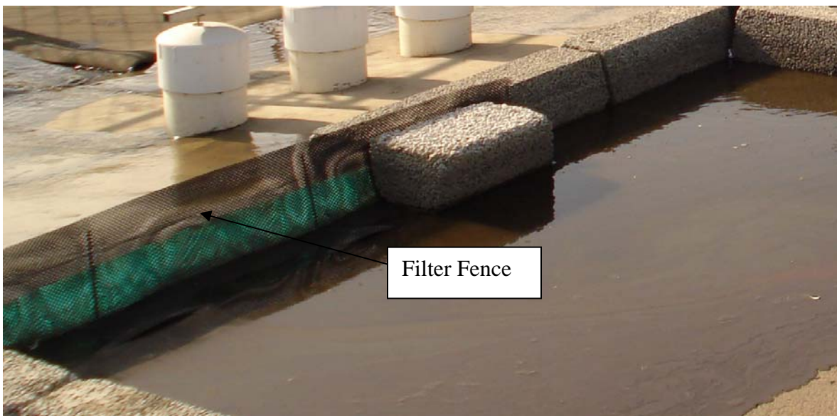
Figure 9. Porous Curb and Filter Fence used for Debris and Sediment Removal.
