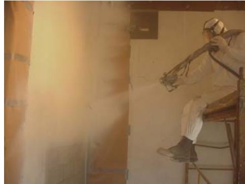
Fig. 1. Application of spray-on polymer
