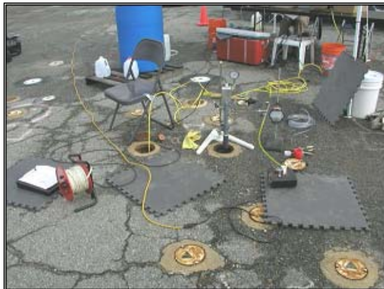
Figure 3-13. Pump Test Setup
