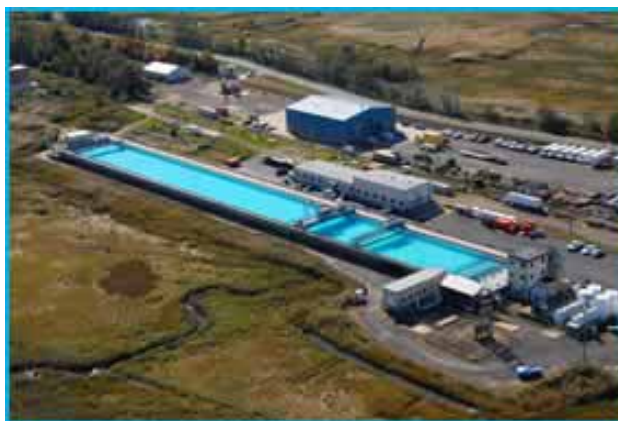
Figure 1. OHMSETT test facility.
