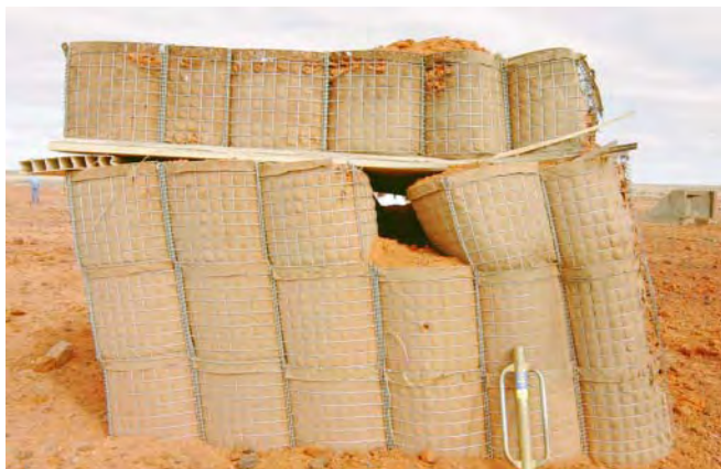
Figure 2. Heavily damaged but stable structure
