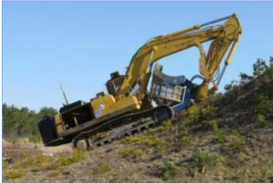
Figure 11: CAT 325 Excavator with Sifter Bucket
