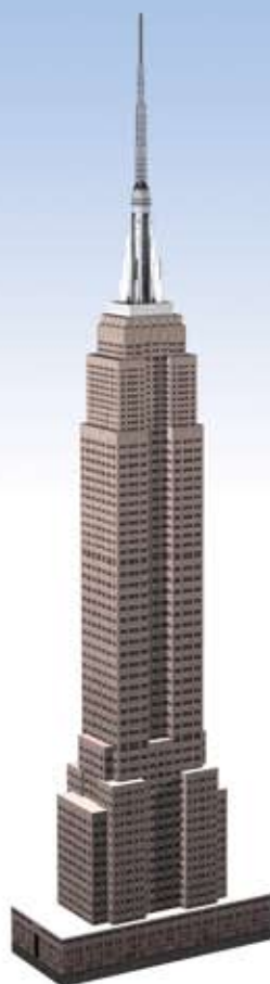
Empire State Building 1,454 ft
