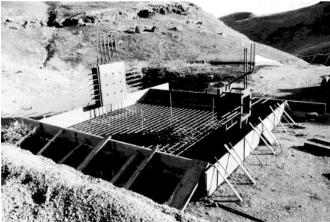
Figure 7. Early construction, showing embedments for the door (left) and bullnose (right).
