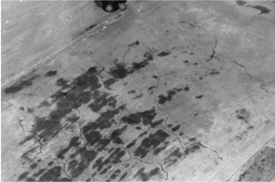
Figure 23. Interior cracks in floor between anvil and north wall.
