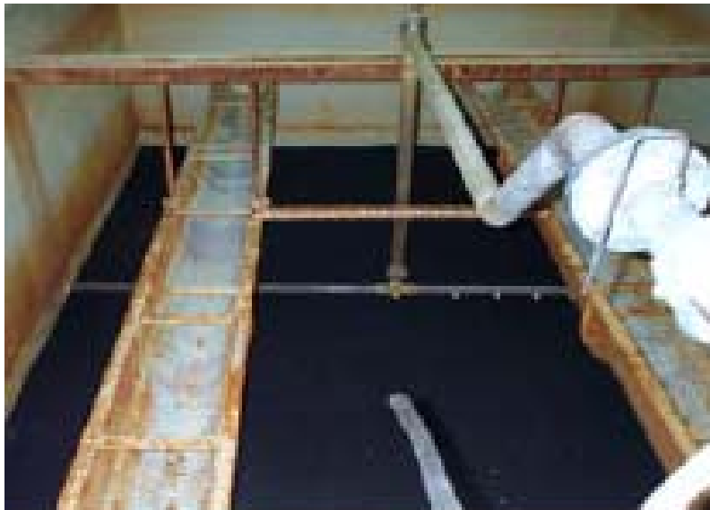
Figure 3a. Metal troughs and wash piping in single filter cells before coating refurbishment.
