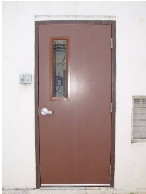
Figure 11b. Typical steel door at chlorine building at wastewater treatment plant after refurbishment.
