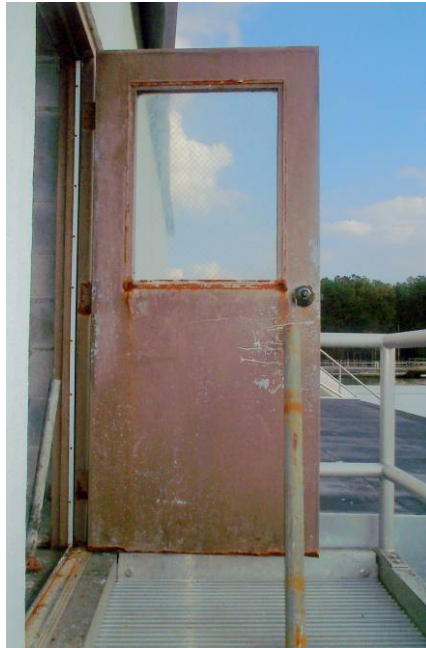
Figure 11a. Typical steel door at chlorine building at wastewater treatment plant before refurbishment.
