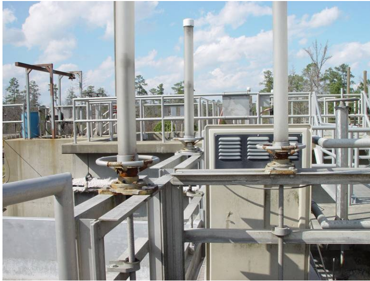
Figure 12a. Severely corroded (un-salvageable) corroded steel hand wheels at WWTP before replacement.
