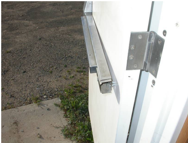
Figure 17. Screws attaching the panic bar to the door shown in Figure 16 showing that the door has bent and pulled the screws from the door.
