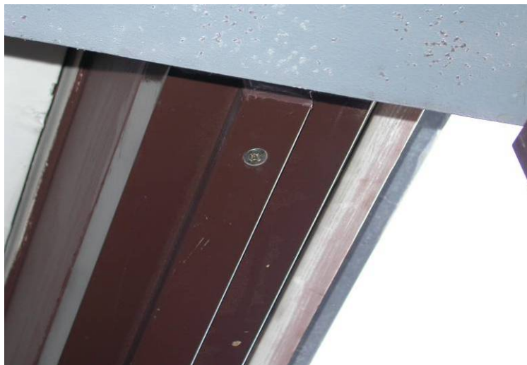
Figure 9. Overhead door sill cut to allow equipment loading track shown in Figure 8.
