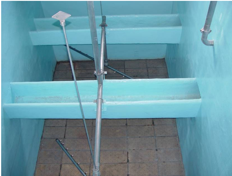
Figure 2b. Concrete surface in dual cell water filter after refurbishment.
