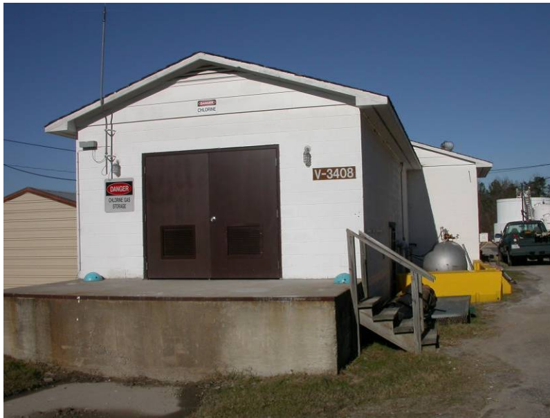
Figure 5. Replacement doors for the doors shown in Figures 1–3 above.
