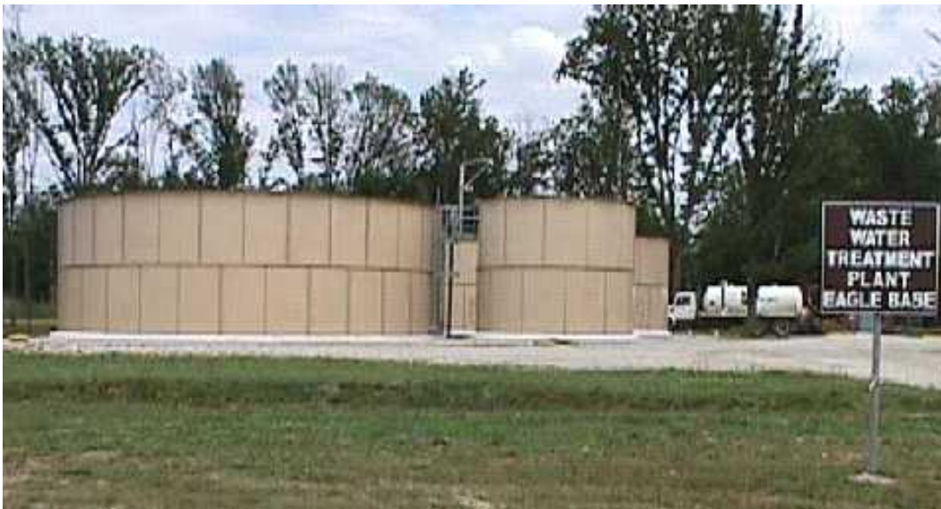
Figure E6. Sequencing batch reactor (SBR) and sludge tanks for brigade-size base camp.p.
