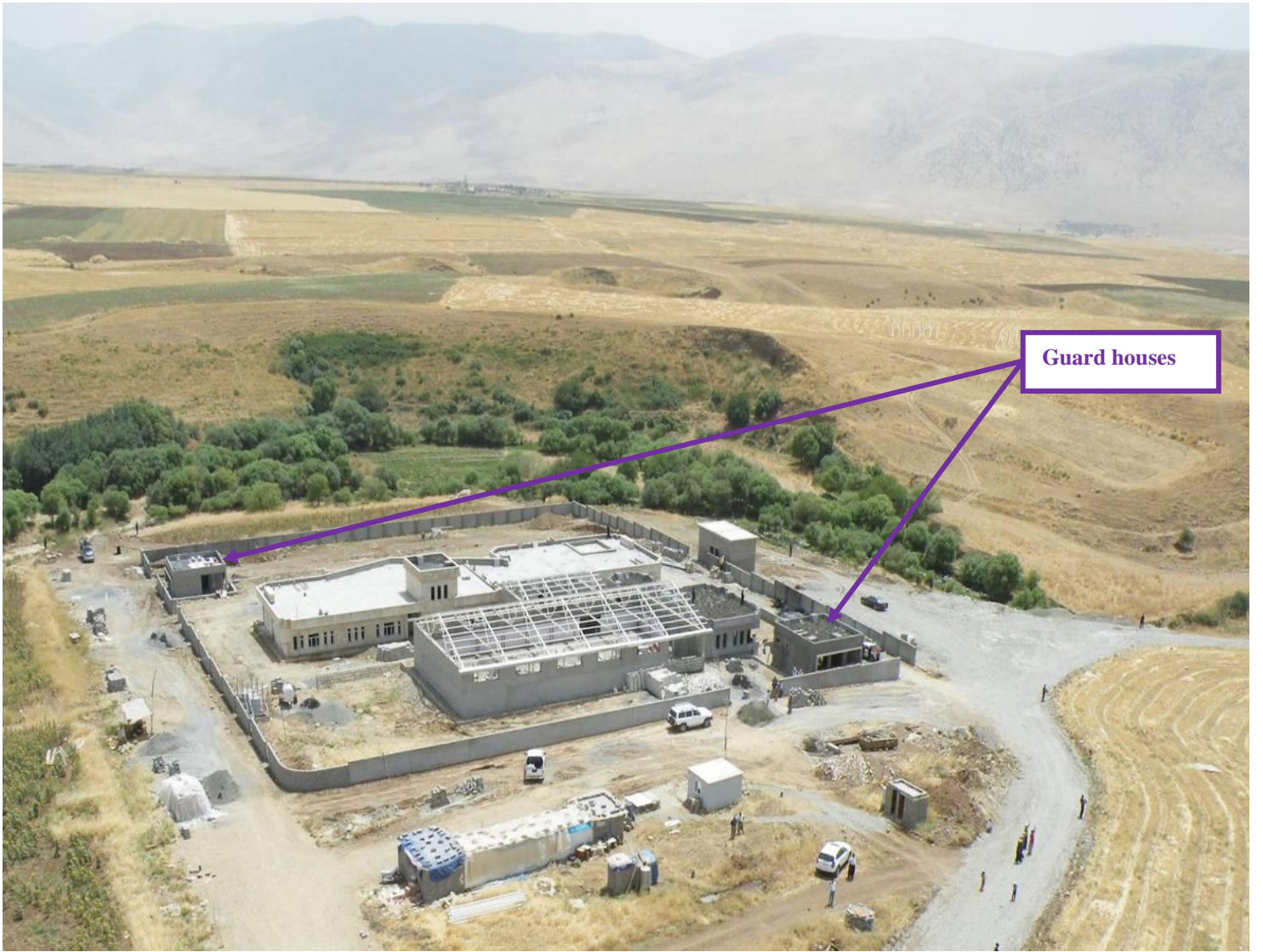
Site Photo 6. Location of the guard houses within the abattoir facility
