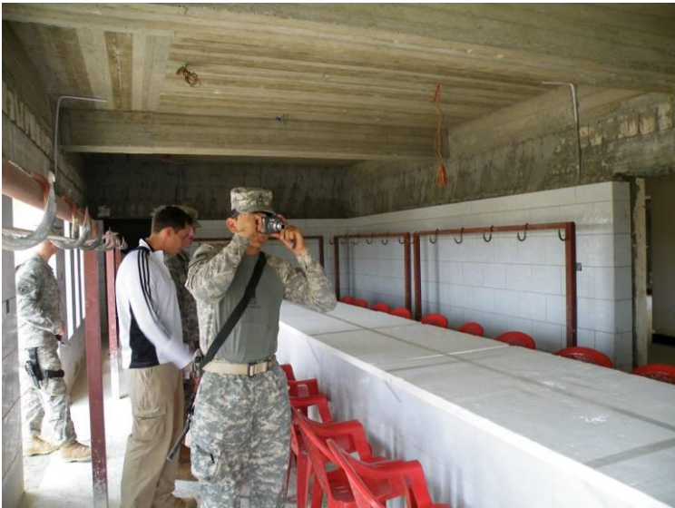
Site Photo 14. View of partially completed meat-testing hall
