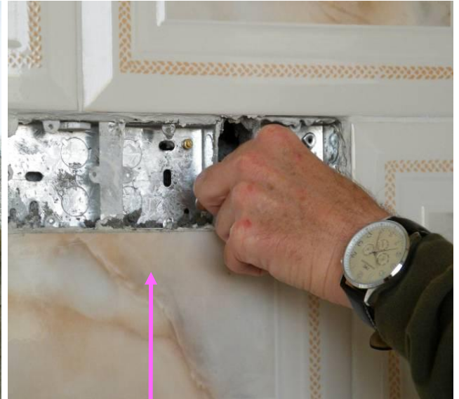
Site Photo 8. Preliminary electrical wiring
