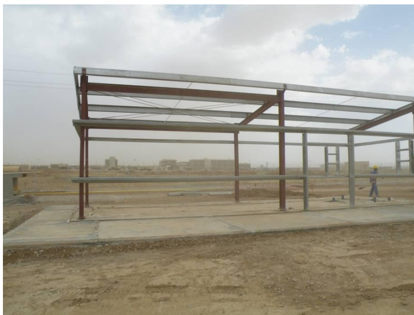
Site Photo 9. Office building
