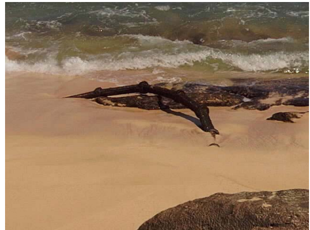
Figure 2. Exposed Split Pipe.
