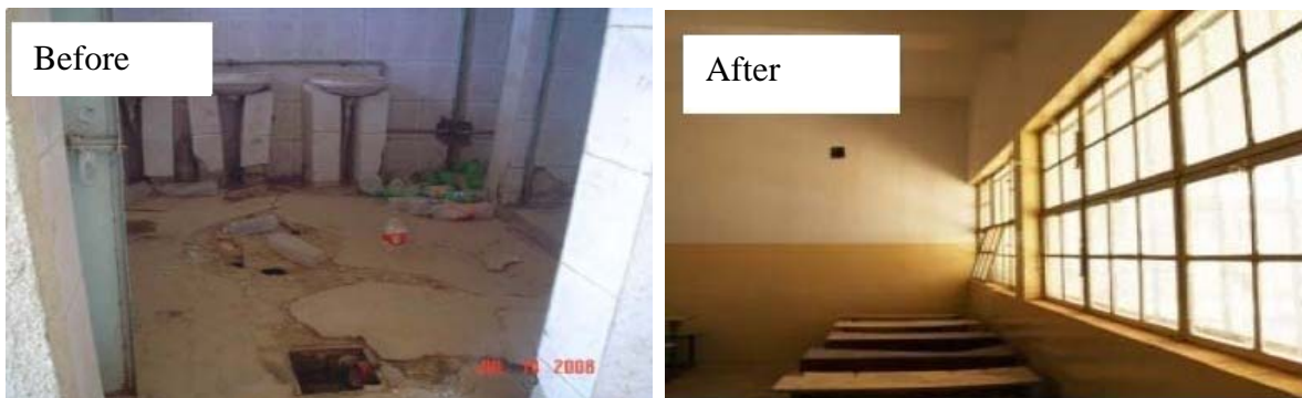
Figure 2—Al Nahreen School Refurbishment
