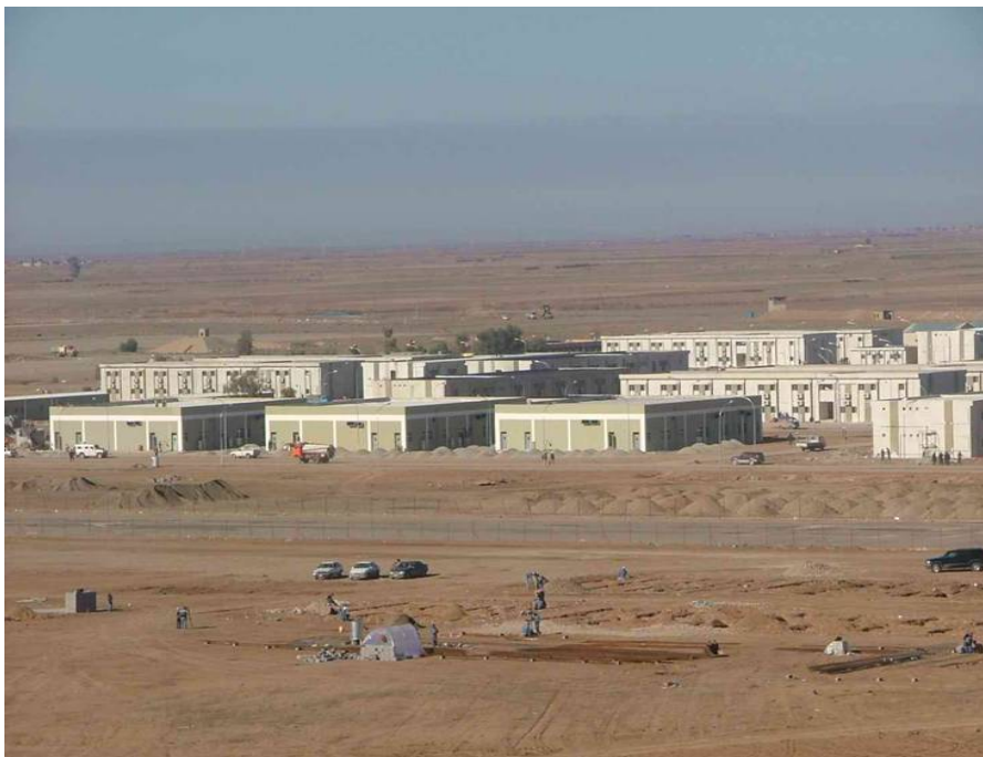
Figure 2—Construction under Two Task Orders at Kirkuk Military Base (December 2004)
