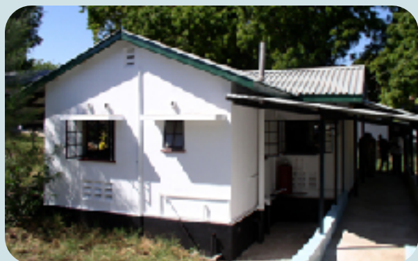
The new facility
